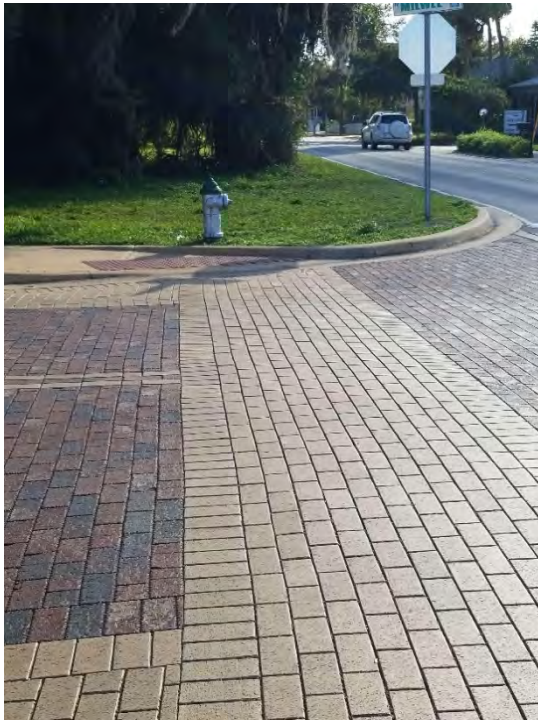
Figure 23: Existing Brick Paver Crosswalk at Milwee Street
