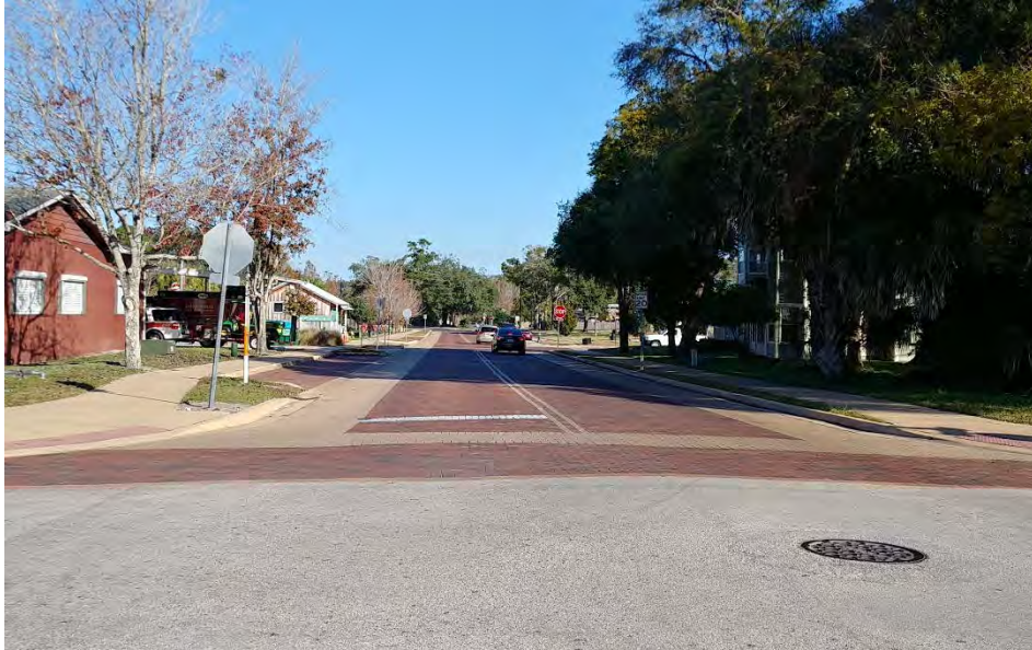
Figure 22: Brick Paver Bicycle Lanes along Milwee Street
